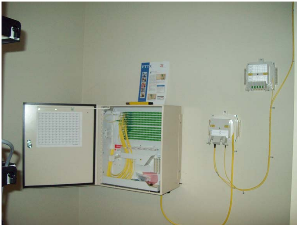
Figure 3 – Spooled Plug and Play Hub, Combiner, and Terminal
